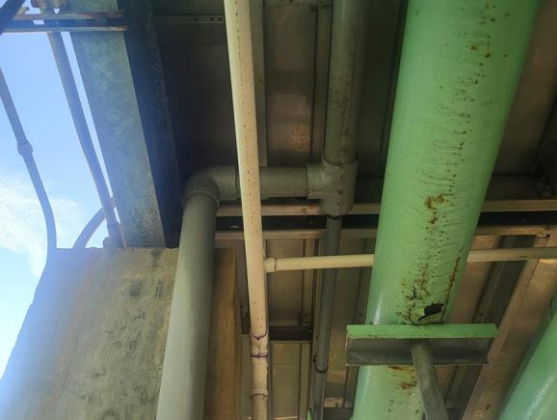
city water station piping to the towers
